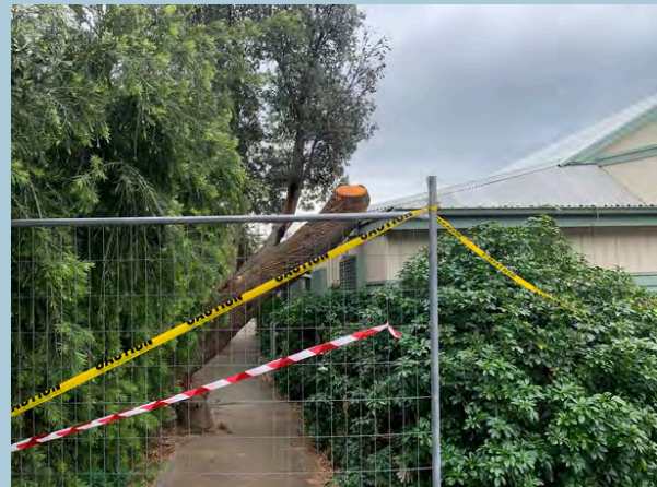
Hastings Hall after fallen tree
